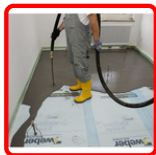
Internal dry area
