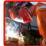
Welding P rotection
